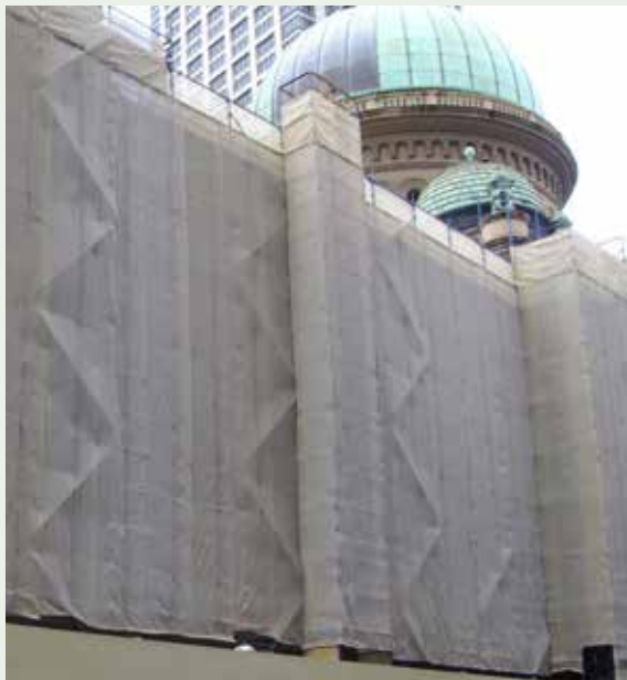
Figure 4.4: The preferred colour for scaffolding mesh is black although for older buildings, including heritage-listed buildings, other colours that are sympathetic to the building and locality may be required.
