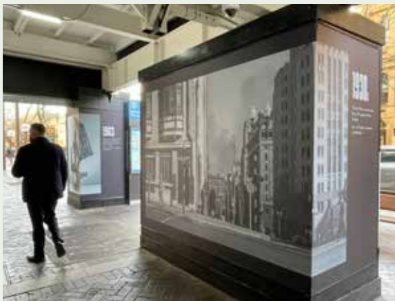
Figure 3.38: Counterweights exceeding the prescribed maximum dimensions including height must be fully enclosed and graphics displayed on all surfaces. The top image shows large counterweights prior to enclosure and the bottom image shows a properly enclosed counterweight.
