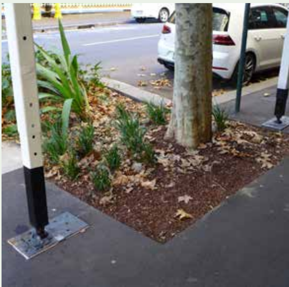
Figure 3.69: The positioning of support columns must accommodate street trees including minimum setbacks from trunks, roots and tree pits. Street gardens must also be maintained (kept clean and tidy) for the full period of installation.
