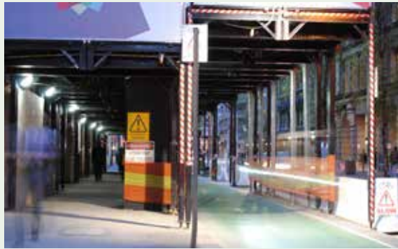
Figure 3.61: Lighting systems over a cycleway must meet a greater illumination standard than that applying to footways .
