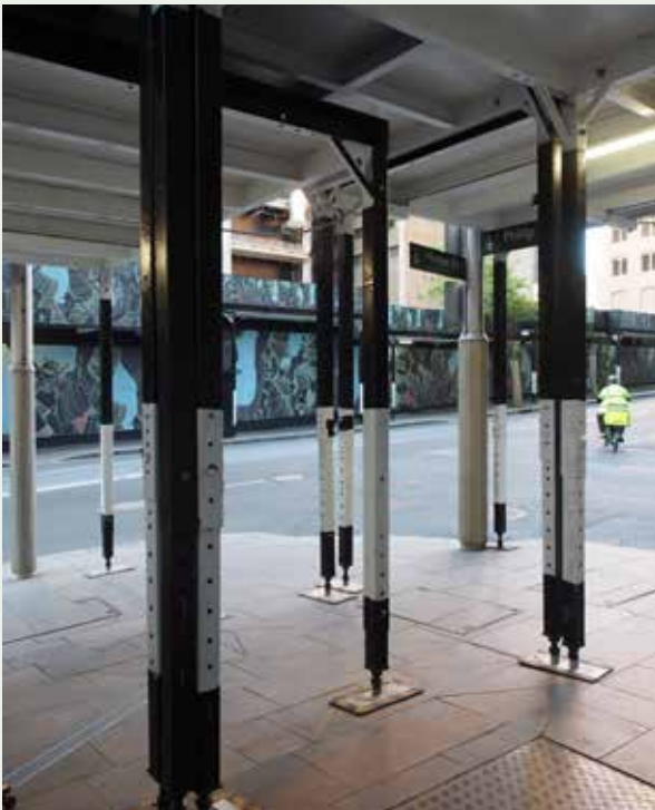
Figure 3.9: Appropriate hoarding column positioning on private land at junction/s with a public footway is important to ensure safe, convenient and accessible movement of people. This must be considered as part of the hoarding design process.
