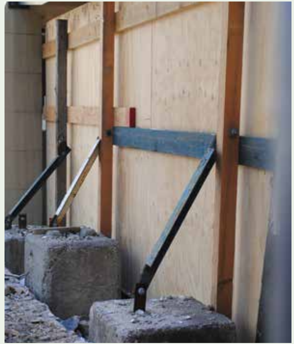
Figure 3.37: Typical concrete block counterweight with lateral bracings.
