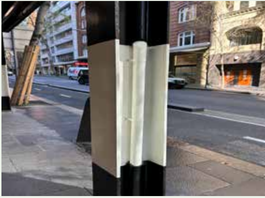
Figure 3.49: Deck drainage pipes must be attached to columns and painted to match the column.*
