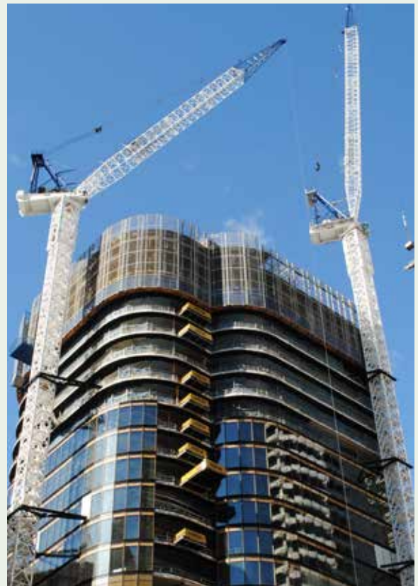
Figure 1.2: Approval is required when swinging or hoisting material over a public road or slewing any part of a crane over a road including vaning actions. Refer to the City's 'Code of Practice: Hoisting and Construction Activities On and Above Roads' for further information.
