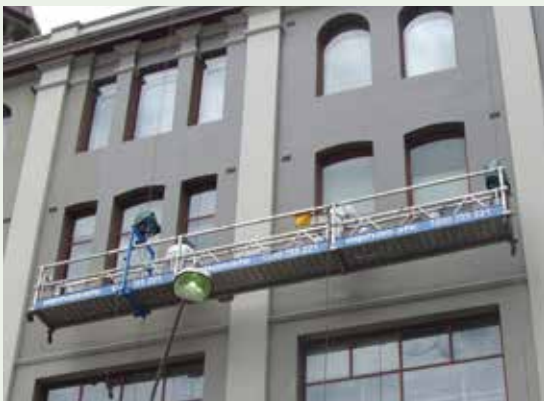
Figure 3.51: Suspended scaffolds (swing-stages) require approval for both use and parking/placement on a hoarding deck.*
