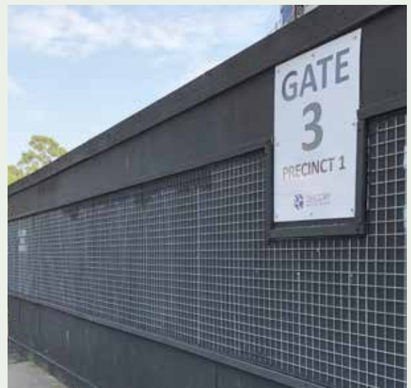
Figure 3.47: For problematic sites in the non-city-centre area that are regularly impacted by bill poster attachment, the display of graphics in accordance with Part 06 may be necessary. Alternatively, meshing of site fences may be permitted subject to meeting minimum prescribed standards and obtaining the approval of the City .
