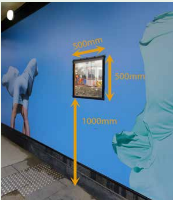
Figure 3.46: Where sites are to be excavated deeper than 1.5m viewing windows for the public must be provided in the site fence at the required dimensions, height and number.
