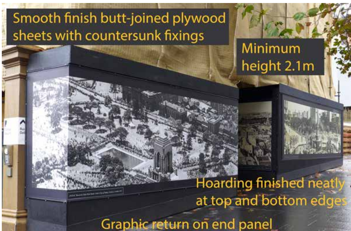
Figure 3.44: A typical Type-A hoarding . All surfaces must be painted black and the top and bottom of the fence capped and trimmed. Graphics must be displayed where required by Table 1 in Part 06 .
