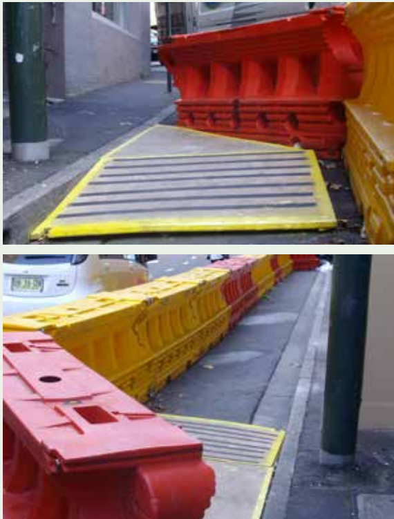
Figure 3.42: Where it is not feasible or practicable to keep a footway open, particularly in cases where narrow footways will be impacted, temporary pedestrian pathways and kerb ramps may be used where the roadway has sufficient width to safely accommodate the encroachment (temporary pathway). This design solution must be endorsed by the City's Traffic Operations Unit.
