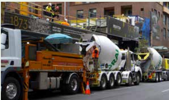
Figure 2.5: A hoarding approval (permit) does not include an approval to use the roadway for the loading and unloading of building material and equipment. A separate approval must be obtained (refer to the 'Code of Practice: Hoisting and Construction Activities On and Above Roads' for further details).
