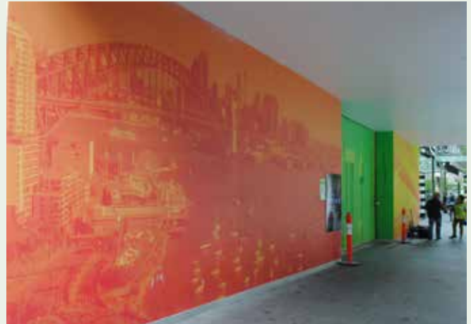
Figure 3.52: Fully lined hoarding soffits are permitted subject to mandatory six-monthly inspection by a structural engineer able to be undertaken.*
