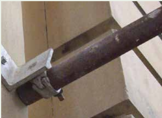
Figure 4.3: Scaffold fixings to heritage-listed buildings should be avoided but where necessary, comply with the provisions in 4.4.2 .
