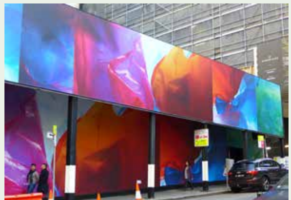
Figure 3.56: A fascia must cover all structural members of custom-built hoardings and any sheds, approved equipment and/or material storage (see 3.13.2(a) ). Note that the fascia of modular gantry systems does not need to screen perimeter beams and knee bracings at column connections.
