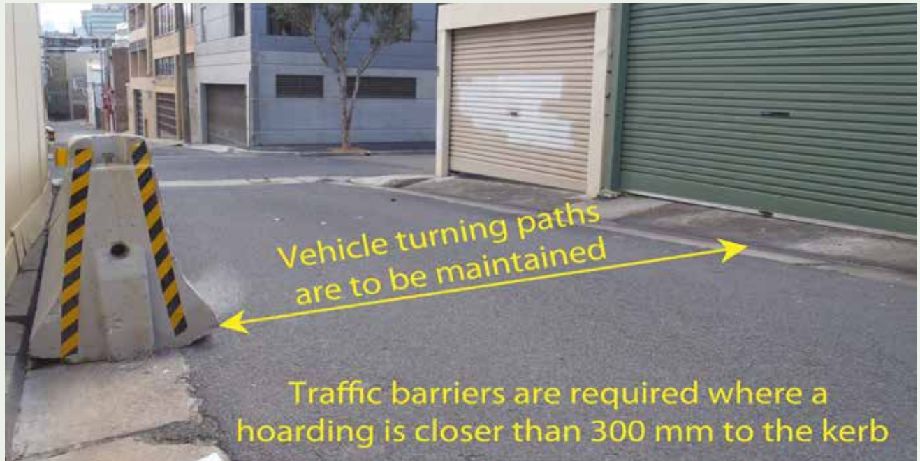
Figure 3.39: Temporary traffic barriers are required where a temporary structure is located within 300mm of the kerb. Where this cannot be achieved, barriers placed in the kerb gutter may be permitted where there are no impacts on turning and manoeuvring pathways at vehicle crossings and entrances to properties/garages. Applicants will need to verify compliant vehicle turning paths using swept-path diagrams templates (refer to AS/NZS 2890.1).
