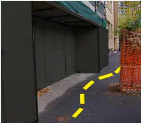
Figure 3.40: Where hoardings are erected on narrow footways it may be necessary to indent hoarding fences and scaffolding (using ladder beams) to provide clear minimum widths around infrastructure (signage stems, parking ticket machines, light poles etc.) and street trees . A clear height of at least 2.4m must be provided in the recessed sections.
