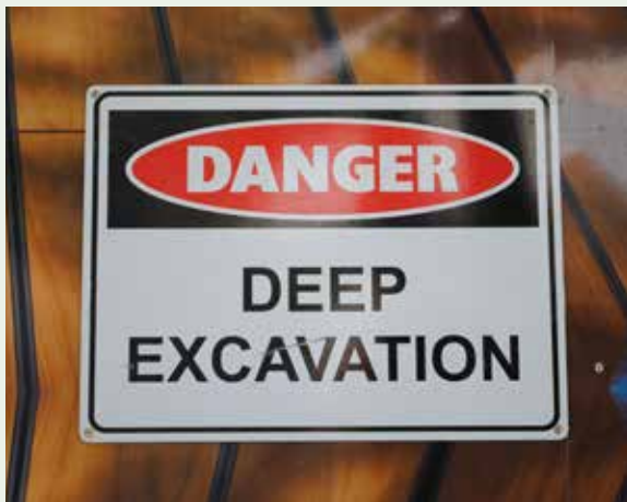
Figure 2.15: For hoardings associated with an excavated site (deeper than 1.5m), caution signage must be displayed indicating a deep excavation behind the site fence. Signage should be appropriately positioned to avoid placement over graphics (see Part 06 ).
