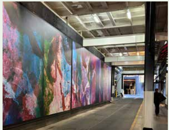
Figure 2.20: When planning to place a hoarding over a laneway special design considerations must be given to the potential impacts on surrounding buildings and occupants including fire-related aspects (see 2.14 ). Consultation with likely affected parties must also be undertaken.
