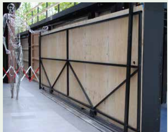
Figure 3.58: Large access doors/gates in site fences must be adequately framed, finished and supported. Doors, hinges and roller systems including connections must be specified, checked and certified by the design engineer.
