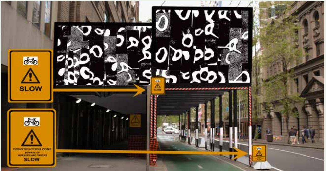
Figure 3.27(a): Type-B hoardings erected over cycleways must satisfy special design and operational requirements including caution signage and distinctive markings on columns at the portals.
