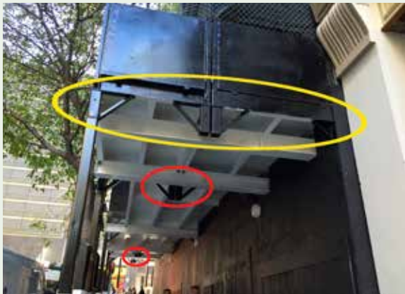
Figure 3.57: Example of a non-compliant design. Fascias must extend to cover the structural members in a single plane to allow graphics to extend over the entire surface (circled yellow). Note also that all structural members to the soffit of the deck are to be painted white.
