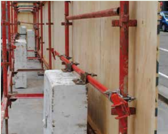
Figure 4.8: Scaffolding encapsulating a building undergoing demolition and later used as a hoarding site fence must be adequately counterweighted. Wind actions in the locality including potential extreme wind velocities from surrounding buildings must be considered by the person in control of a worksite and the scaffolding contractor. Excavated sites must also be protected using appropriate pedestrian and traffic barriers (see 2.13).
