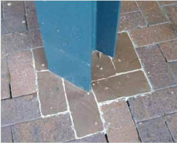
Figure 3.20: The use of fixed columns on footings placed within a footway is generally not allowed. Where there are clearly demonstrated site-specific needs for concrete footings, approval (through lodgement of a road opening application) may be given, subject to stringent design and removal requirements (see 3.8.5 ).
