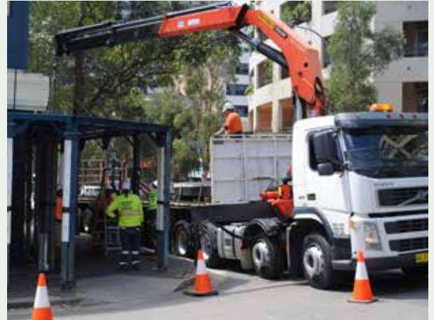
Figure 2.4: The installation and removal of a temporary structure must be undertaken in accordance with the conditions of approval and be continuous once work commences (see 2.11.2(b) ). This includes maintaining safe passage for pedestrians, cyclists and traffic past the area.
