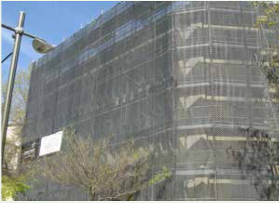
Figure 2.10: The preferred finish for scaffolding is black mesh installed on the outer surface (see Part 04 for further details).
