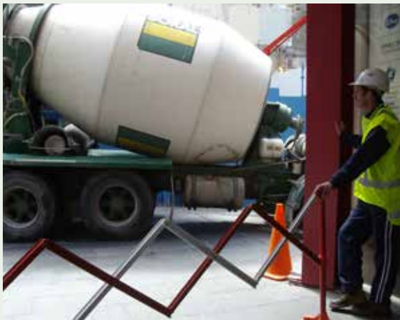
Figure 3.59: Concertina gates to control pedestrian and cyclist movement at truck access points are mandatory in the city-centre and in other busy pedestrian areas outside the city-centre. Gates must be provided on each side of vehicular crossings including cycleways . Specific approval of the City must be obtained before installation/usage.
