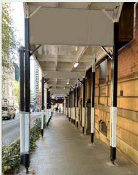
Figure 3.50: Hoardings on sloping sites that need to be stepped with the gradient of the footway must have the vertical openings infilled using 17mm thick structural plywood. The infill panels must be painted to match the white deck soffit.*
