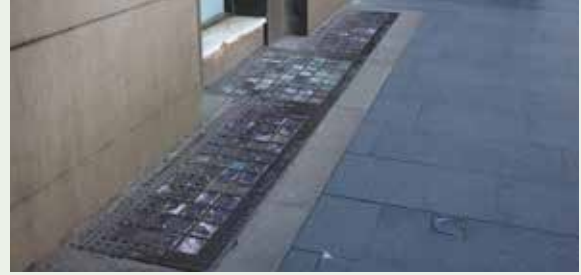
Figure 3.10: Glazed pavement lights provide natural light to basements of older buildings. They are a significant historic feature and must be protected. Column positioning must address setbacks from pavement lights and consider potential basement voids beneath the footway (for adequate bearing capability).
