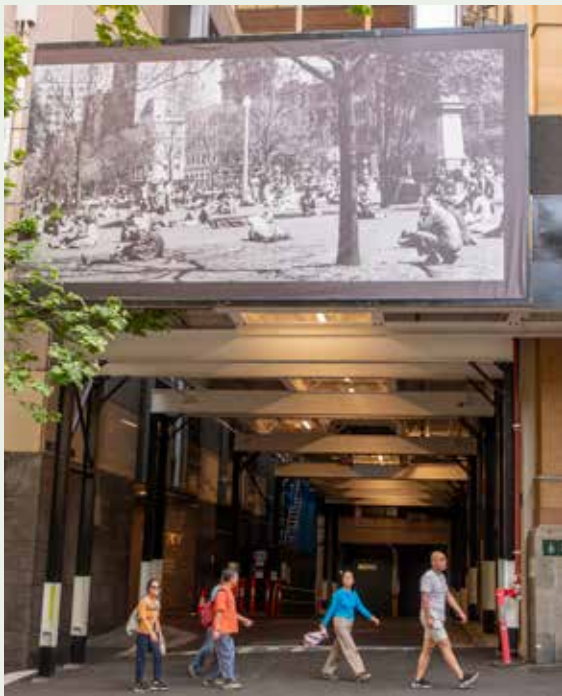
Figure 3.48: When placing a hoarding over a laneway special design considerations must be given to the potential impacts on surrounding buildings and occupants including fire-related aspects. Consultation with likely affected parties must also be undertaken (see 2.14 and 2.15 for further details).
