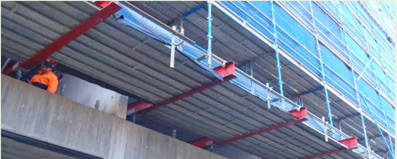
Figure 4.2: Cantilevered work platforms and scaffolding are generally not allowed. In narrow laneways where traffic and pedestrian movement must be maintained, approval may be given subject to systems being fully engineered and certified (see 2.8). Note: Externally installed black screening mesh is the preferred finish (see 4.4.3(e)).
