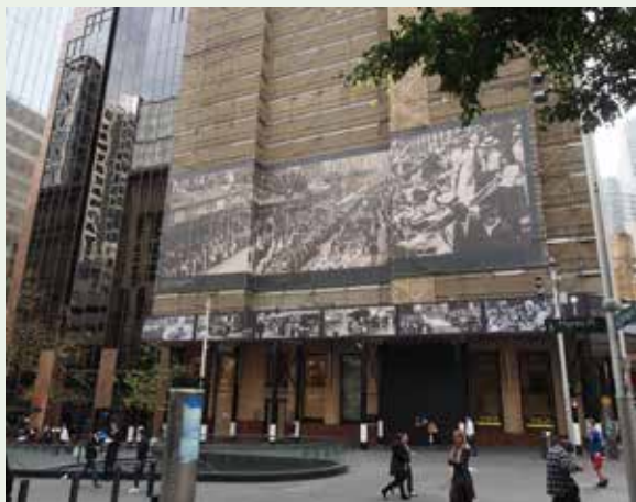
Figure 6.6: Scaffold installation in prominent and highly visible localities may require scaffold wraps (refer to Table 1 ).
