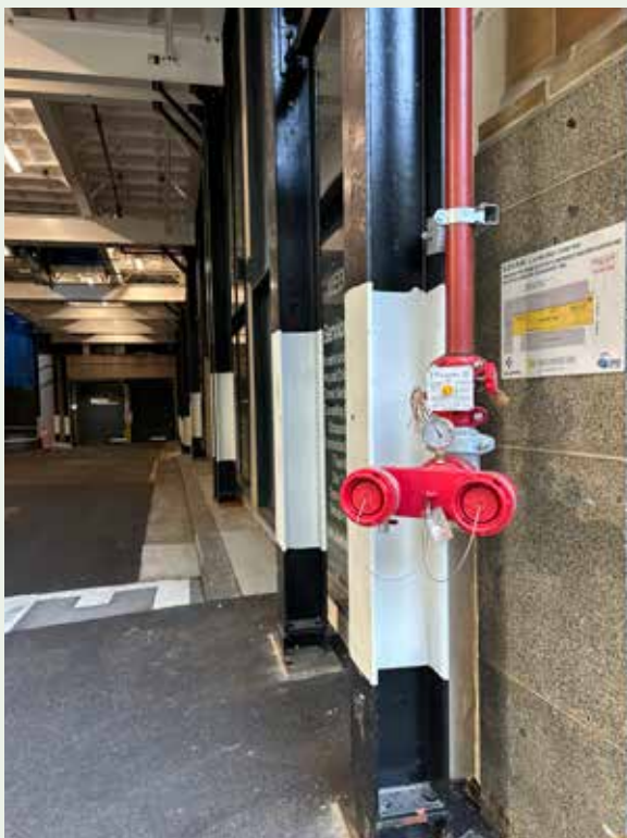
Figure 2.17: Examples of hoardings in laneways with automatic sprinkler protection. The lower image shows a booster connection at the junction of a laneway with a primary road.
