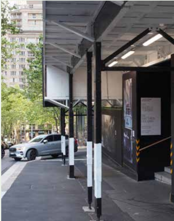
Figure 3.17: The use of cantilevered deck extensions along busy kerblines particularly at bus-stops can assist in minimising column obstructions and reduce impacts on commuter loading and unloading.
