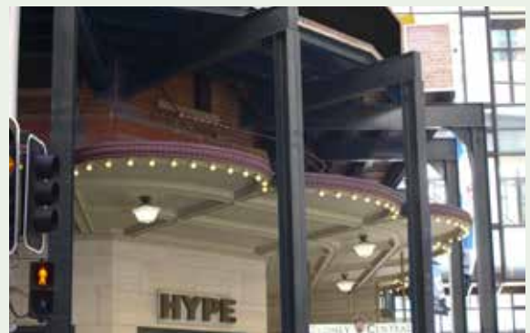
Figure 3.12: Consideration will be given to allow reduced column spacings in the city-centre where there are special needs such as undertaking work on heritage-listed buildings that have significant street awnings that cannot be altered to accommodate column penetrations.
