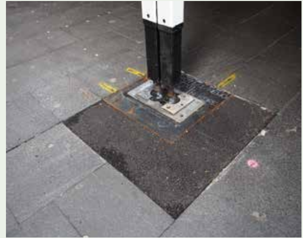
Figure 3.22: Where ground or surface conditions have insufficient bearing capacity to support a temporary structure the City will consider allowing recessed steel plates within the footway subsurface to provide support. Concrete footings may also be considered (see 3.8.5 ). The area surrounding recessed plate/s (or on top of the plate) must be backfilled and evenly finished with material specified and approved by the City . A separate approval ( road opening permit) must be obtained prior to undertaking any work.
