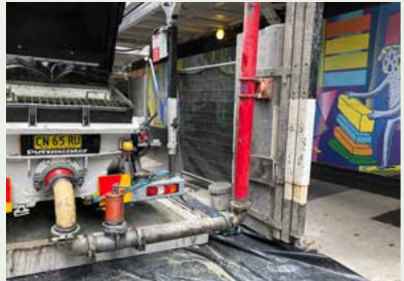
Figure 3.30: Concrete pumping connection points and riser-pipes attached to Type-B hoardings are permitted where an approved works zone is in place on the adjoining roadway and the hoarding is structurally capable of withstanding additional dynamic loads. Permit-holders have work health and safety obligations to protect the public when undertaking pumping operations including complying with SafeWork NSW requirements (see 1.13 for further details).
