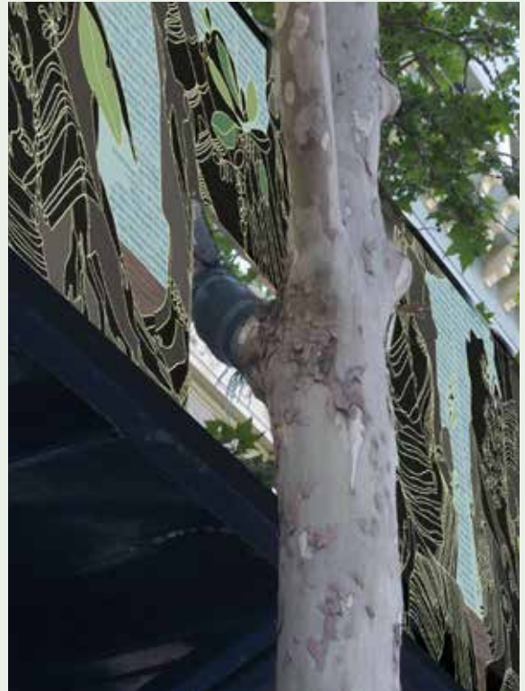
Figure 3.65: Hoardings must be designed to minimise impacts on tree canopies. Penetrations in fascia elements is permitted to accommodate limbs and branches.
