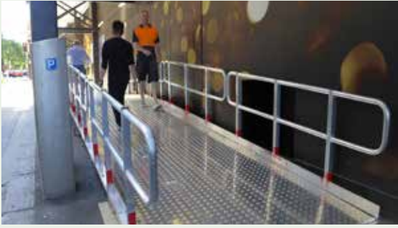
Figure 3.33: Where specific approval is given to install a concrete pumping static-line across a footway , a durable metal pedestrian ramp complying with the minimum design criteria must be provided (see Figure 3.32 ).
