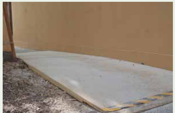
Figure 3.66: Where street tree surface roots are exposed and the use of the tree pit is needed to increase the width of the pedestrian passageway past a hoarding , temporary minor ramping using non-slip plywood sheeting to span over roots may be permitted.
