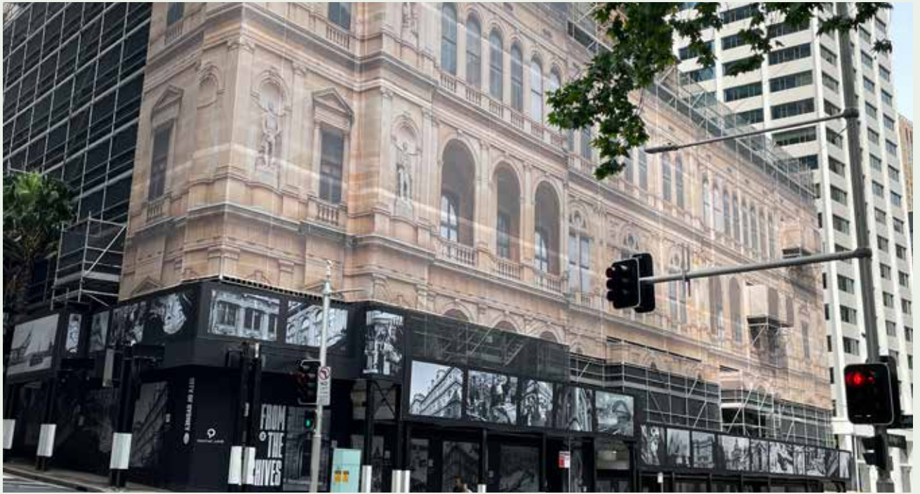
Figure 6.9: An example of a facade replication scaffold wrap on a heritage-listed building.
