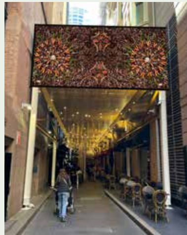
Figure 3.52: Fully lined hoarding soffits are permitted subject to mandatory six-monthly inspection by a structural engineer able to be undertaken.*
