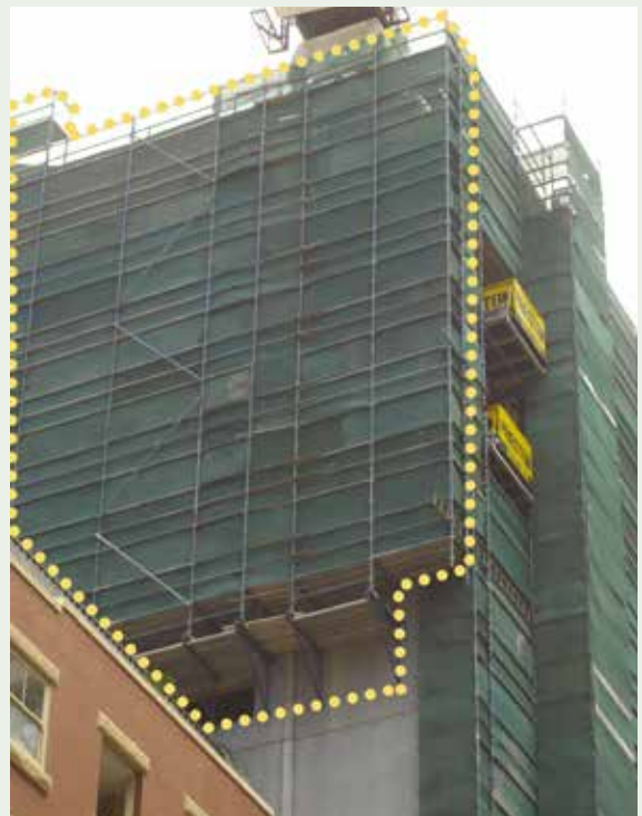
Figure 4.1: Cantilevered work platforms and other temporary structures located over or on private land are not regulated through this Code nor approved by the City . It is the responsibility of the person undertaking the works to obtain an access agreement from affected landowner/s. Access orders under the Access to Neighbouring Land Act 2000 can be sought through the Courts where agreement with neighbouring landowners cannot be obtained.
