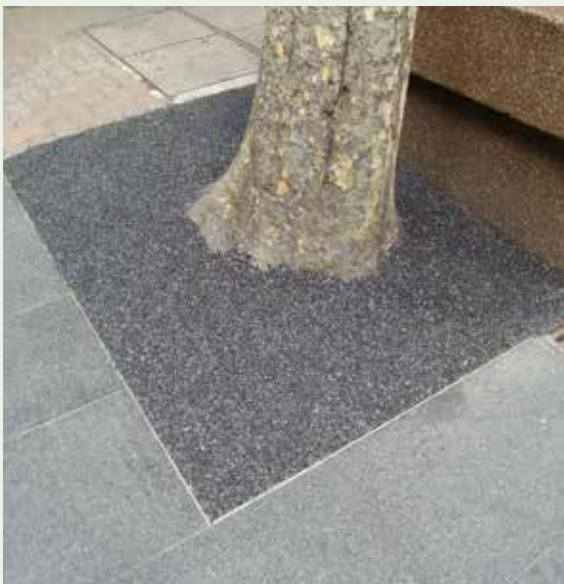
Figure 3.71: Where a temporary structure is in place for a lengthy period (as determined by the City) and there is a need to maximise the available footway width, resin-bonded porous granular paving may be required to stabilise and level tree pits.
