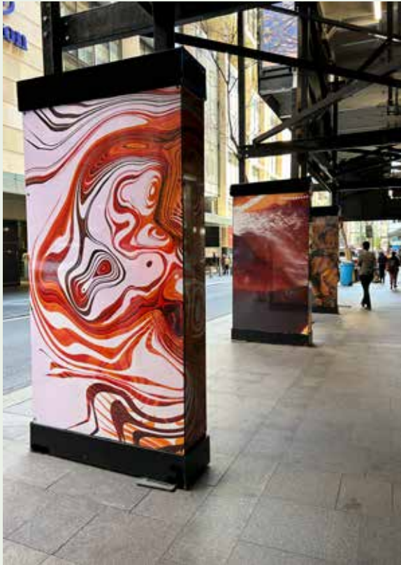
Figure 3.36: Where counterweighting/column placement exceed the prescribed maximum dimensions they must be plywood-sheeted and graphics displayed (see also Figure 3.38 ).
