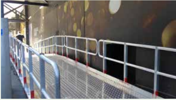
Figure 3.60: In areas of disrupted footway grades such as at truck access crossings and where temporary pedestrian ramps are installed (see Figure 3.32 ), greater illumination intensity must be provided to improve pedestrian safety.
