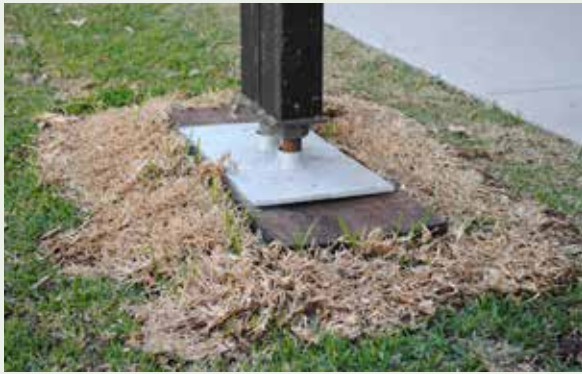
Figure 3.15: The use of hardwood timber soleboards on unsealed ground surfaces to support columns must be assessed and approved by a practising engineer. Soleboards must be periodically checked for continued acceptable durability and stability throughout the installation period. The use of multiple layers of plywood is not permitted. After removal, the nature strip or street garden must be reinstated to a condition acceptable to the City.
